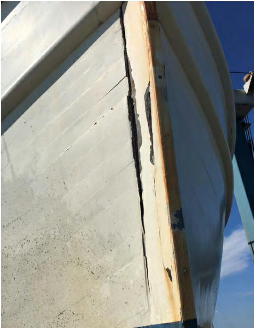
Showing where the hull plank ends have parted from the stem allowing water ingress
